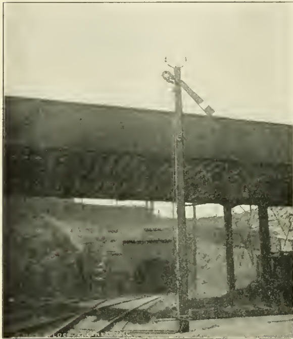
SLOT SIGNAL GOVERNING ENTRANCE TO THE BERGEN TUNNEL, ON THE ERIE.
